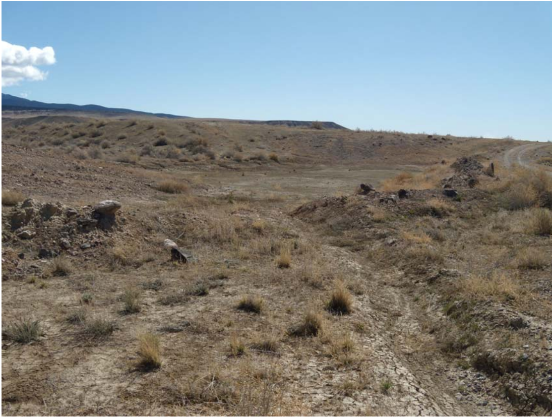
GRJ 3/2011. PL-3. East storm water and sediment collection pond.
