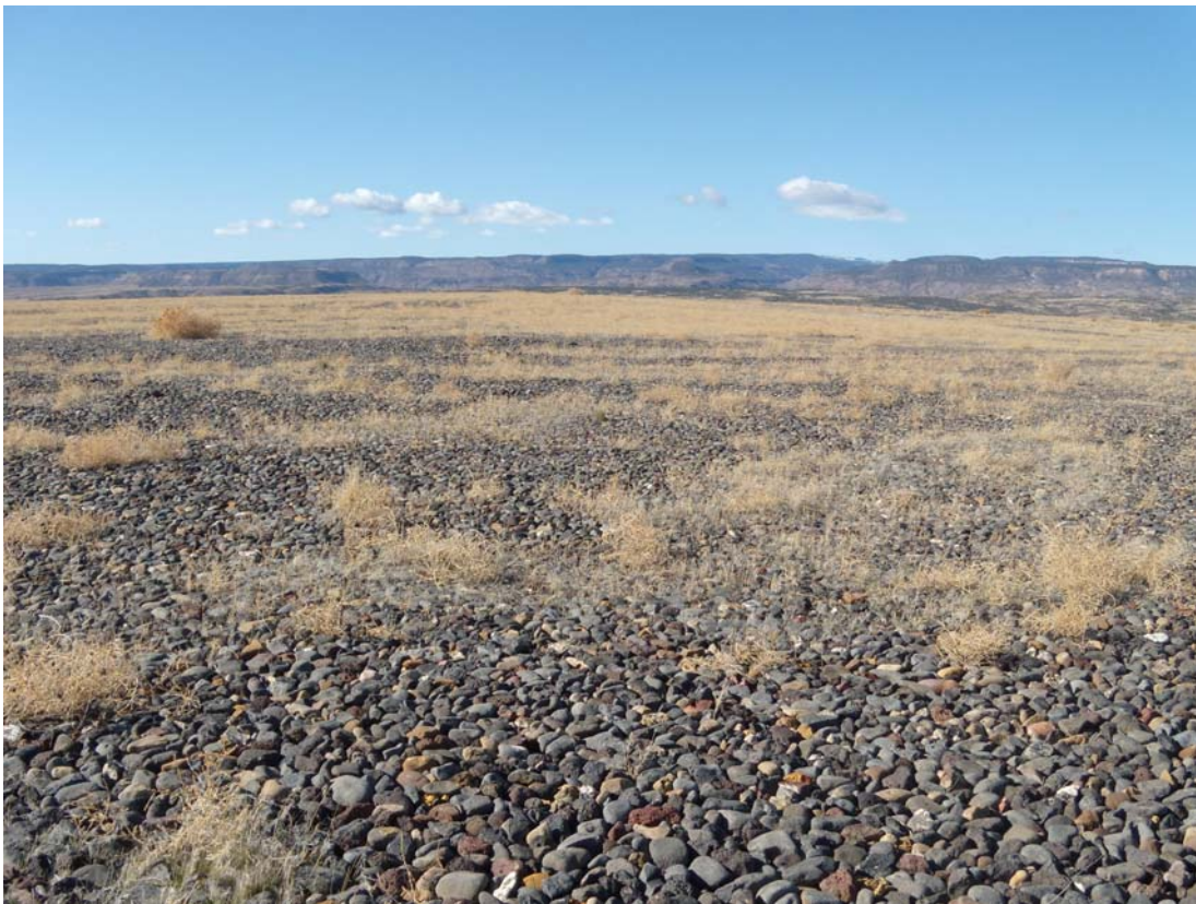
GRJ 3/2011. PL-2. Northeast corner of the disposal cell cover.
