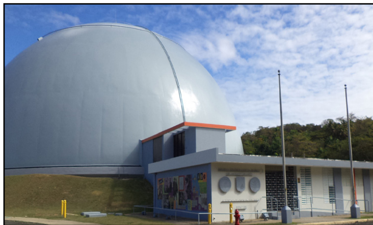
The BONUS Site Reactor Dome Was Repainted in 2014
