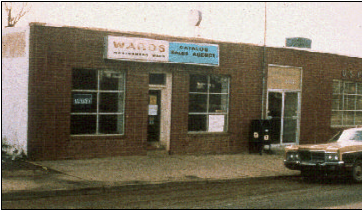
The Montgomery Ward store (shown here) and the Harry Randall house were the first properties remediated under the Monticello Vicinity Properties Project.
