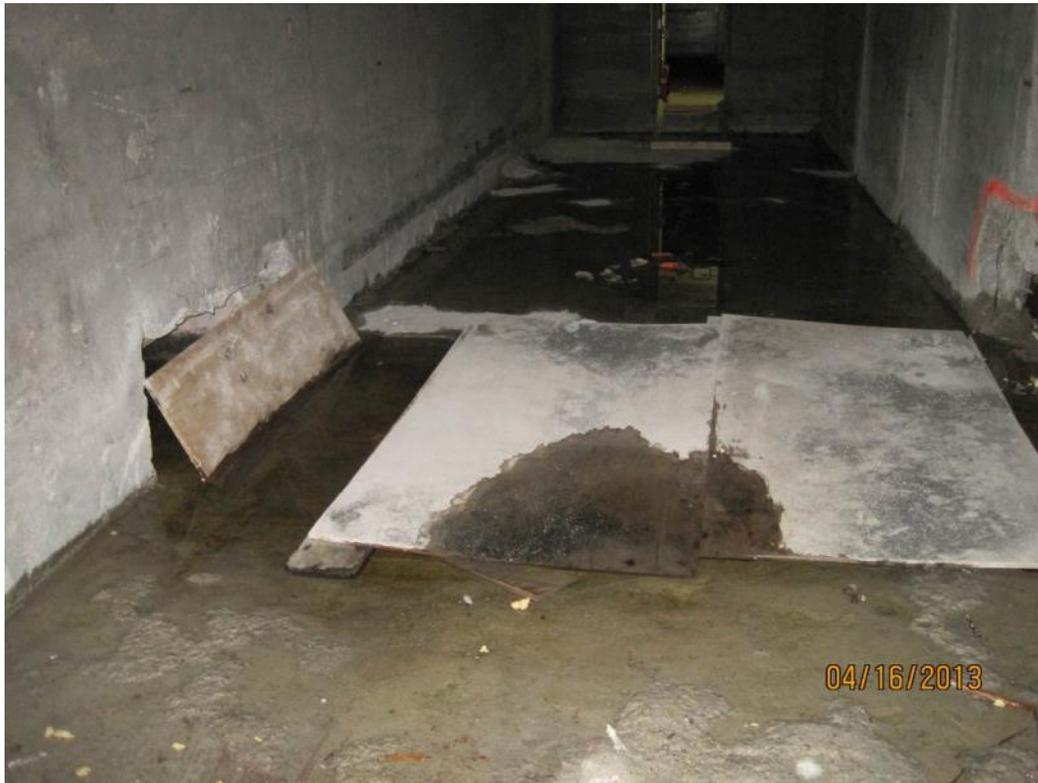
*Figure 18. Standing Water Caused by Sump Pump Failure in T Building Room 57, Observed During the IC Walkdown*
